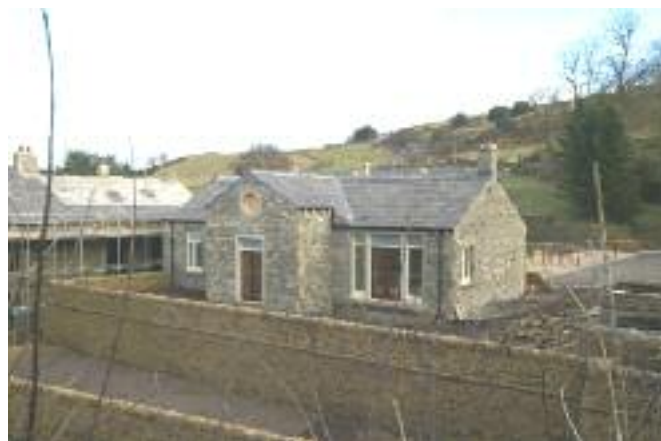
View of the property from over the stream
